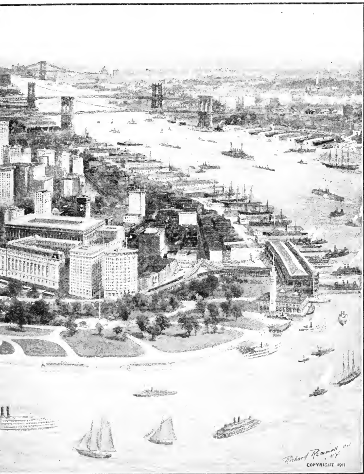
Custom House Bridges Battery Barge Office South Ferry worth two billion dollars, most of them built within a dozen years. Six are ers or agencies of businesses aggregating over $400,000,000,000 of investments.
